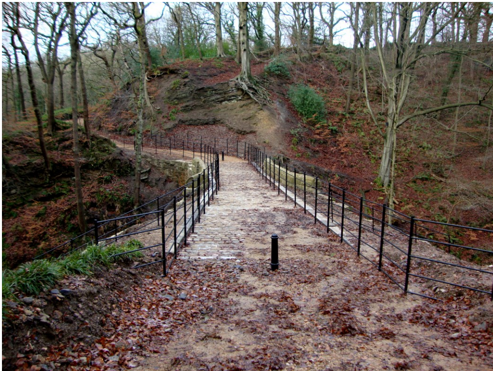
Alum Scar Bridge on the old road from Blackburn to Samlesbury. (Courtesy of L.C.C.)
