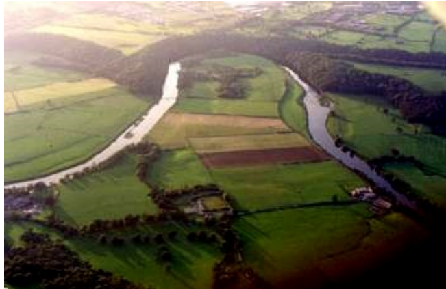
Photo showing Samlesbury Lower Hall and the Grade I/2 Agricultural land within Horseshoe Bend.
